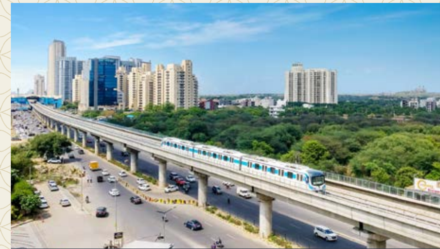
Metro Rail Connectivity - The ultra-modern way
