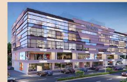
Aruna Arcade, Patancheru
