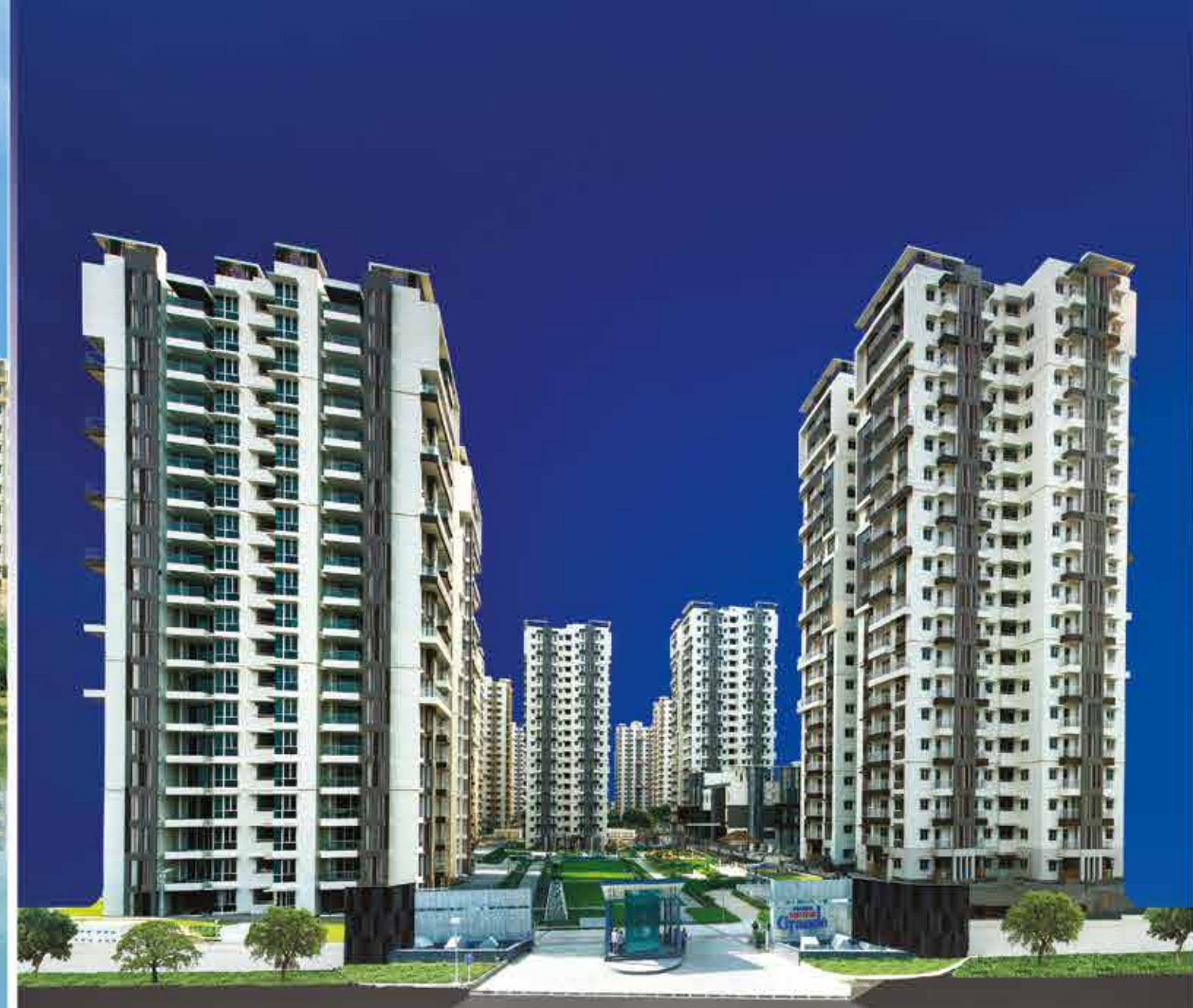
Actual picture shot at location
