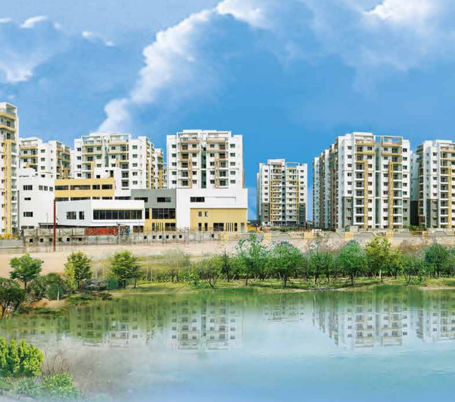
Actual picture shot at location
