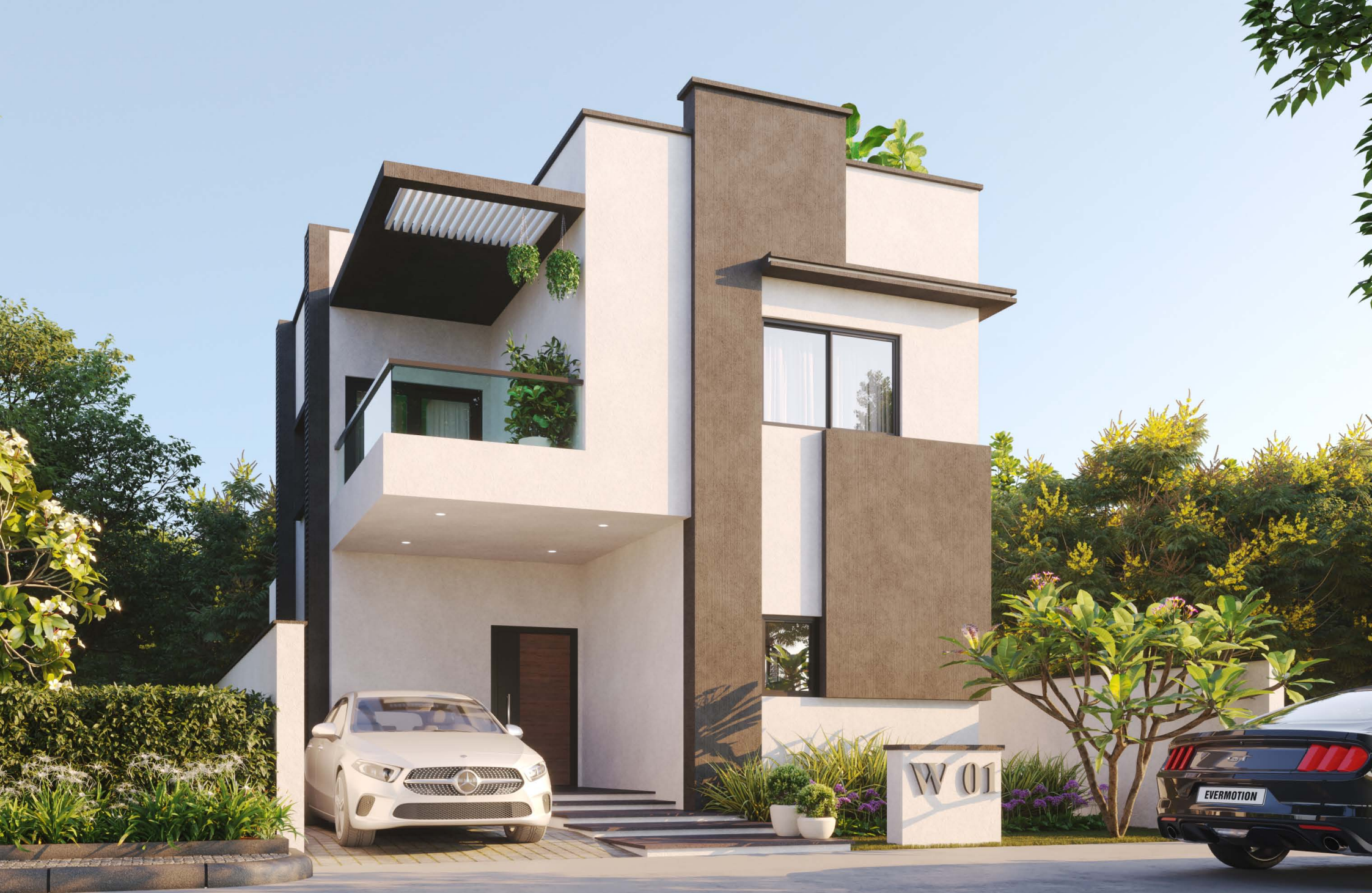
150 West Facing Villa
