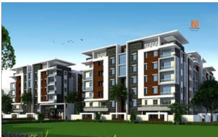
Concrete Melody @ Chandanagar
