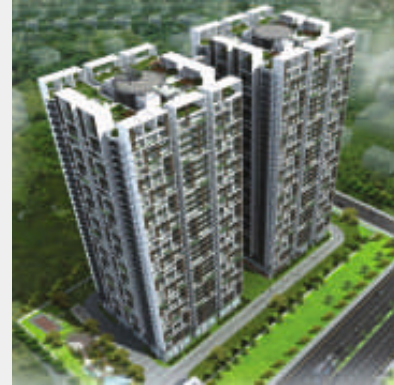
Oxygen Towers (Completed) Seethammadhara
