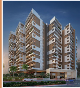
Veda Homes @ Kandanur Near Financial District Exit 12
