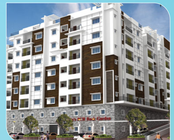
Jains PCH Rock Garden I, II & III Madhapur
