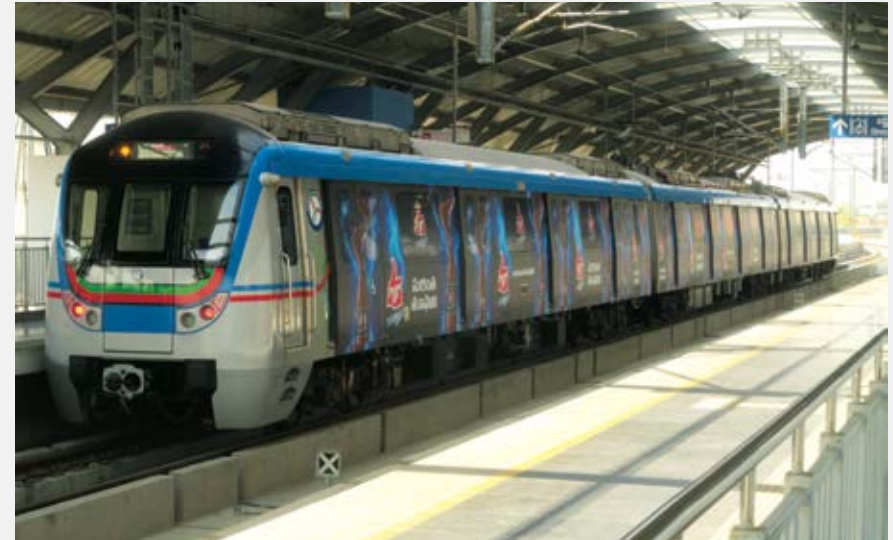
Proposed Elevated Metro High Speed Train between Hyderabad - Vijayawada
