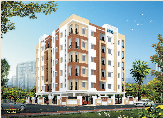
GATEWAY RESIDENCY (20 Flats) Amaravathi Road, Guntur
