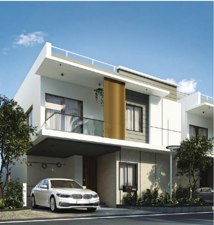
West Facing Villa
