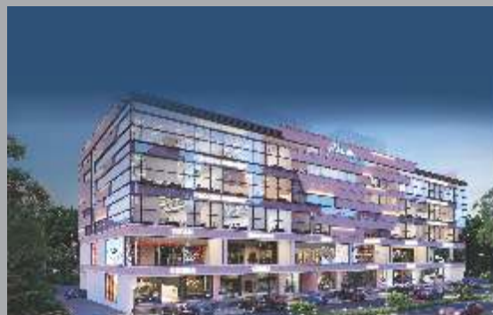
Aruna Arcade, Patancheru
