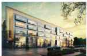
RAICHANDANI MALL Kompally
