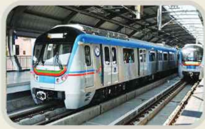
Prop. Hayathnagar Metro Station
