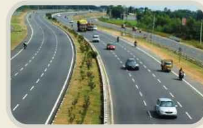
NH 65 Vijayawada Highway
