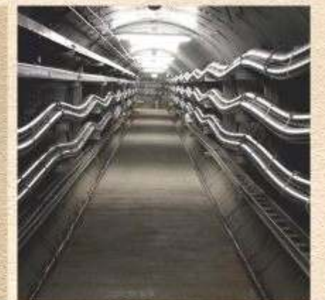
Under Ground Cabling of wire.
