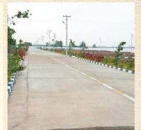
RCC Internal Road with Decorate Street light
